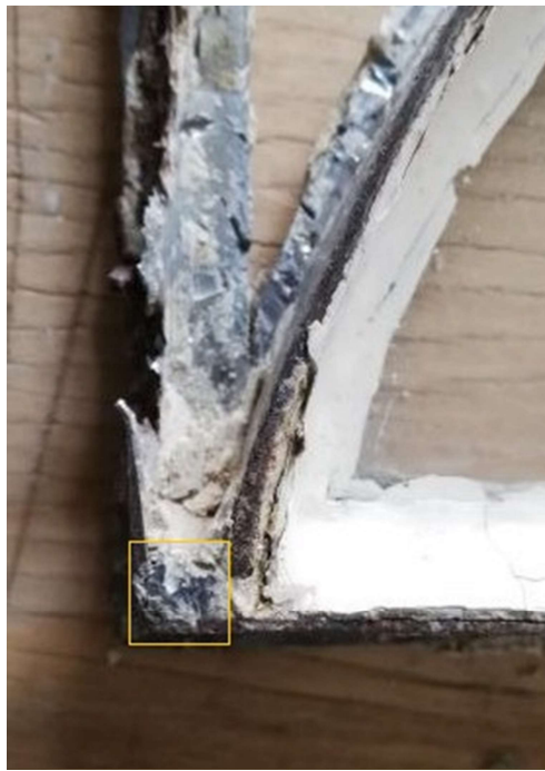
Fig.16 - Solder block in the corner of Casement 1
