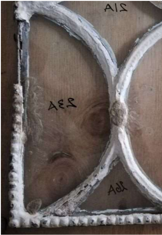
Fig.29 – Missing lead carelessly puttied over, Casement 1
