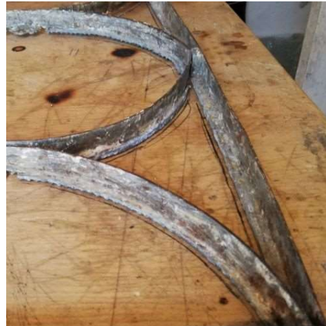
Fig.14 - Patches of orange corrosion, Casement 1
