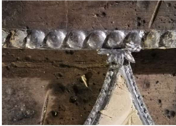
Fig.76 – Cast lead replacements in place, C2
