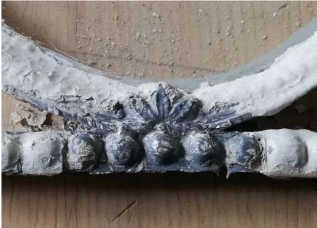
Fig.43 – Removal of paint using UV heat gun detail, Casement1
