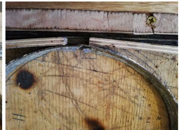
Fig.56 – Preparation for new solder block, Casement 1
