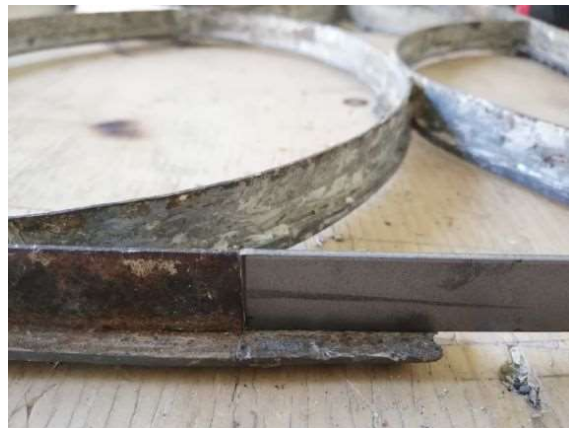
Fig.48 – Smooth join between new metal and original, C1
