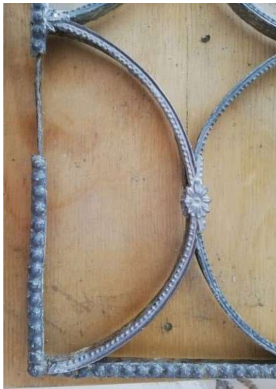
Fig.64 – Replacement decorative lead, Casement 1
