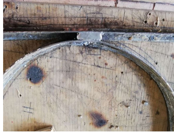
Fig.58 – New solder block, Casement 1
