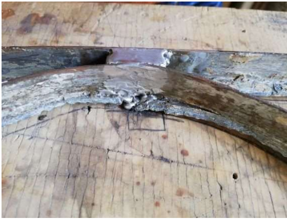
Fig.57 – New solder join, Casement 1
