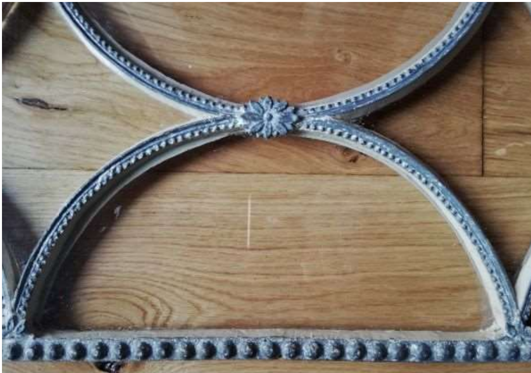
Fig.66 – Lead front was puttied as steeply as possible
