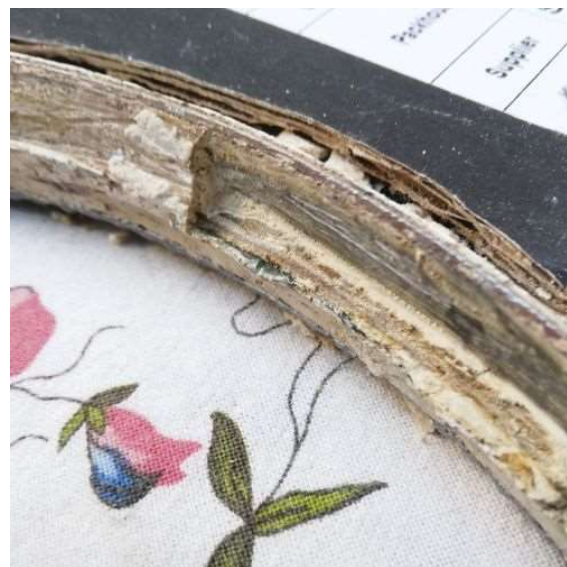
Fig.70 – Retaining variety of depth in bedding putty, C2
